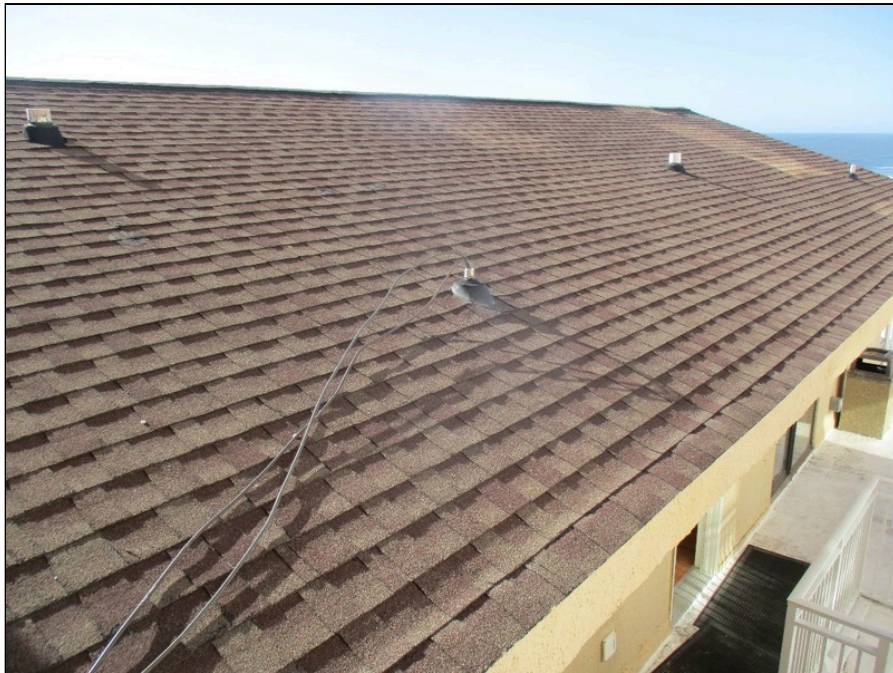
22 - Tides penthouse shingle roof overview
