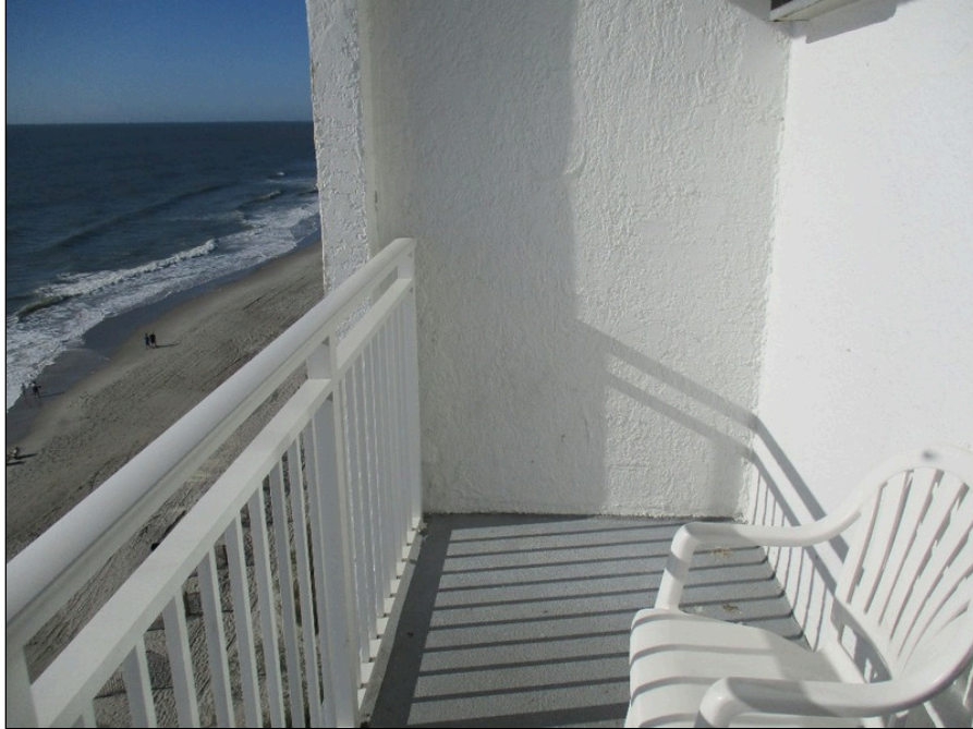
7 - Typical balcony at Tides
