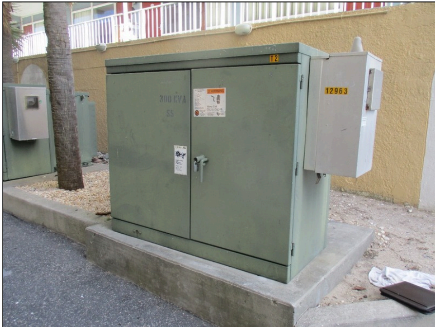
30 - Electrical transformer
