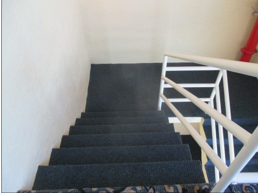
49 - Typical stairway finishes
