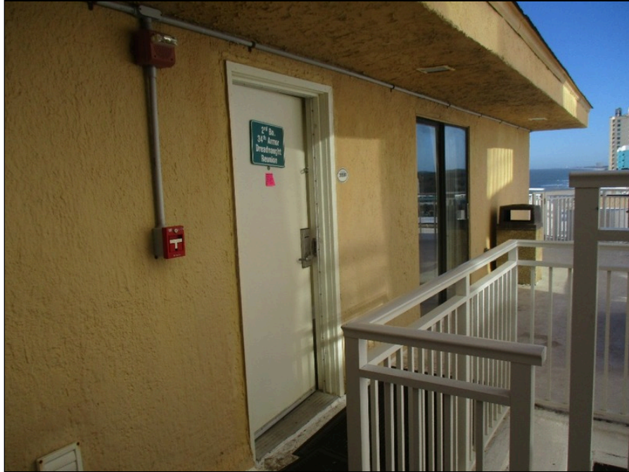
9 - Exterior corridor at Tides penthouse
