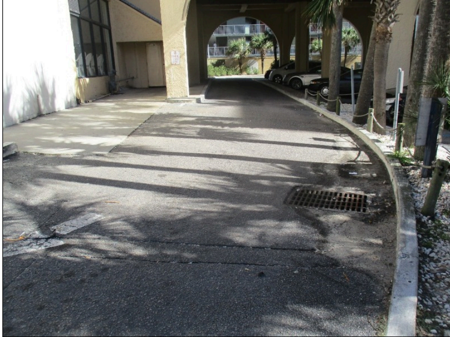
15 - Service drive with drop inlet
