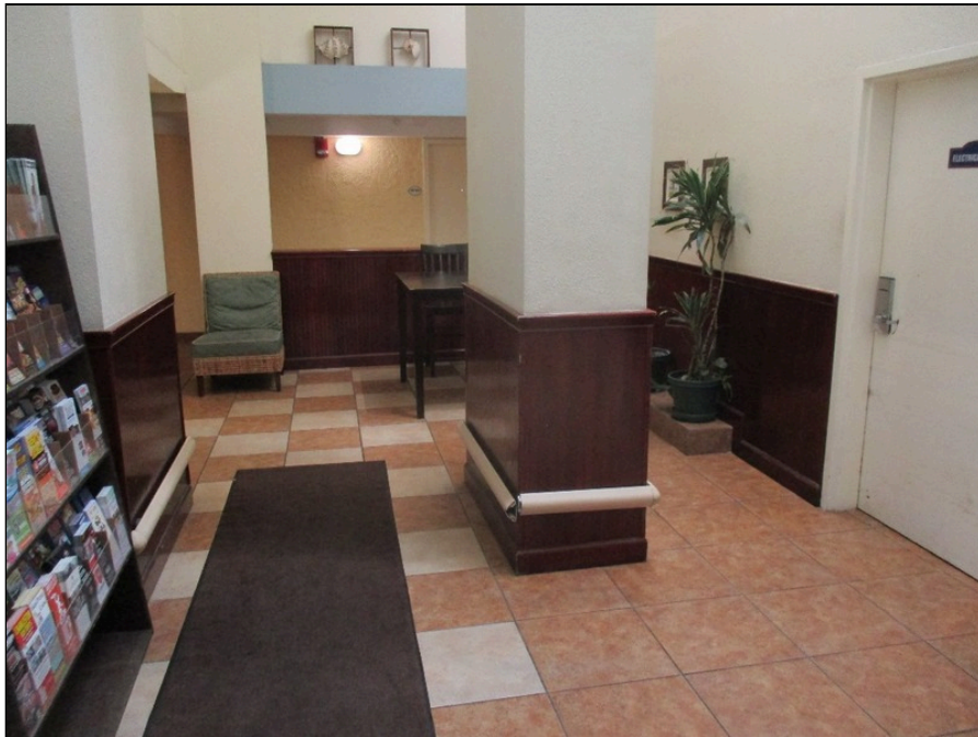
48 - Corridor finishes adjacent to lobby area
