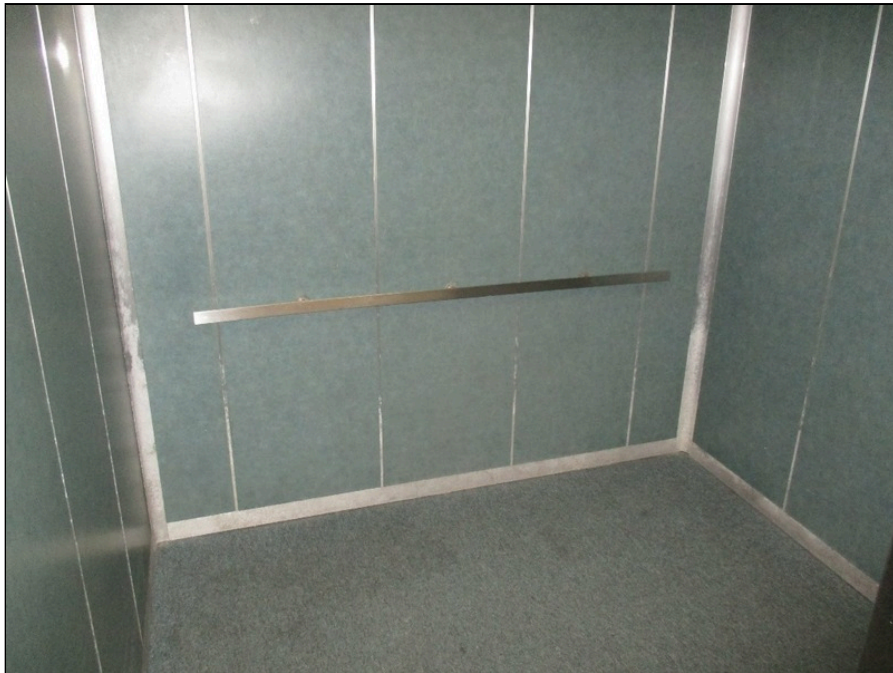
28 - Typical elevator cab finishes
